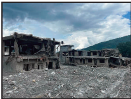
Floodwaters leave a trail of destruction across Nepal
