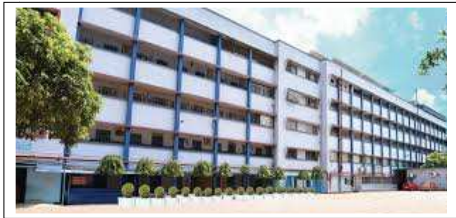
FIG 3.1 Shri Shikshayatan College Building
